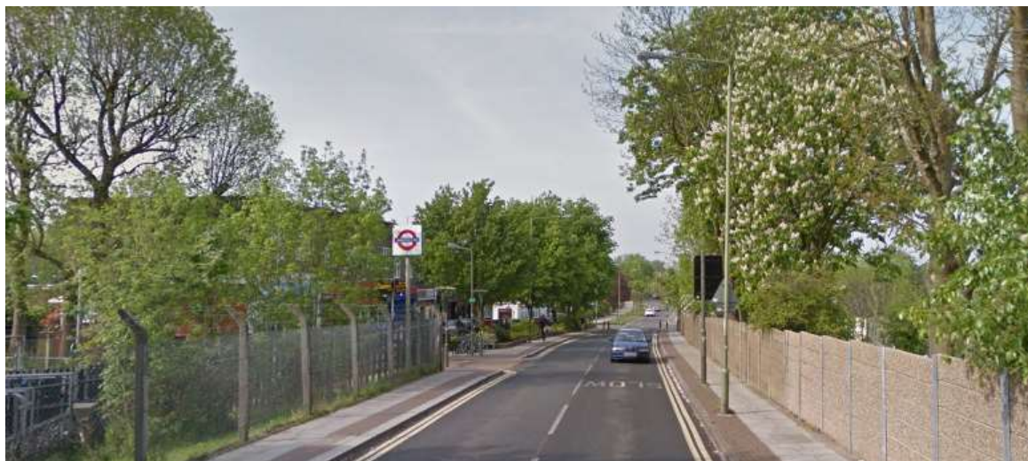
West Finchley station has a poor profile from street level, with a lack wayfinding signing and bus interchange
