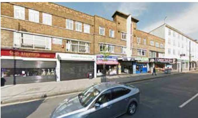
Image 2: street view towards Grand Arcade
