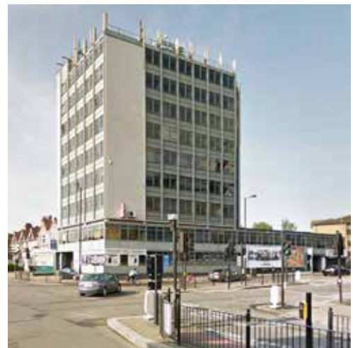
Image 14: street view of existing office building
