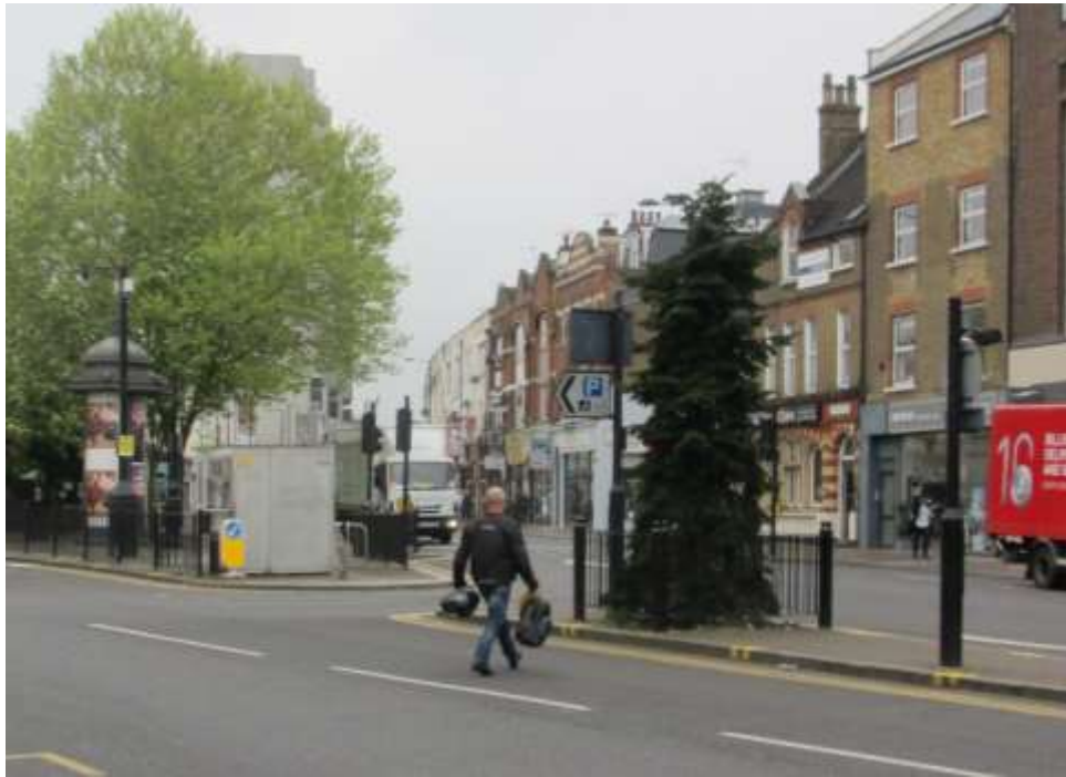
The Existing Situation, Ballard's Lane / High Road junction
