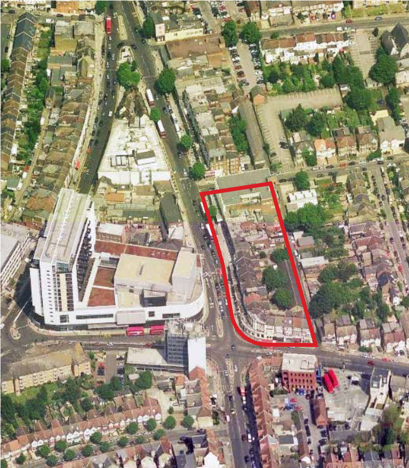
Image 19: existing aerial view of East Wing site
